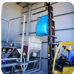
Bulk bags unloading battery
