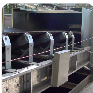
Conveyor belt with belt scale
