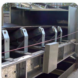
Conveyor belt with belt scale
